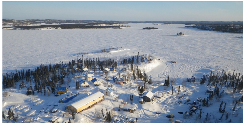
Infrastructure at the Damoti camp and the winter landscape from above.
